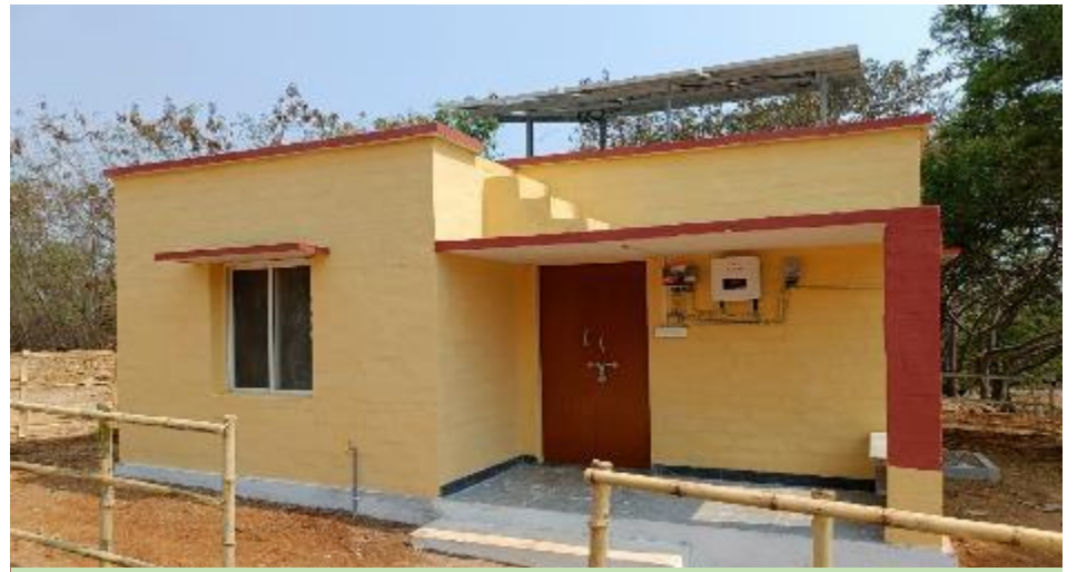
View after completion of painting
