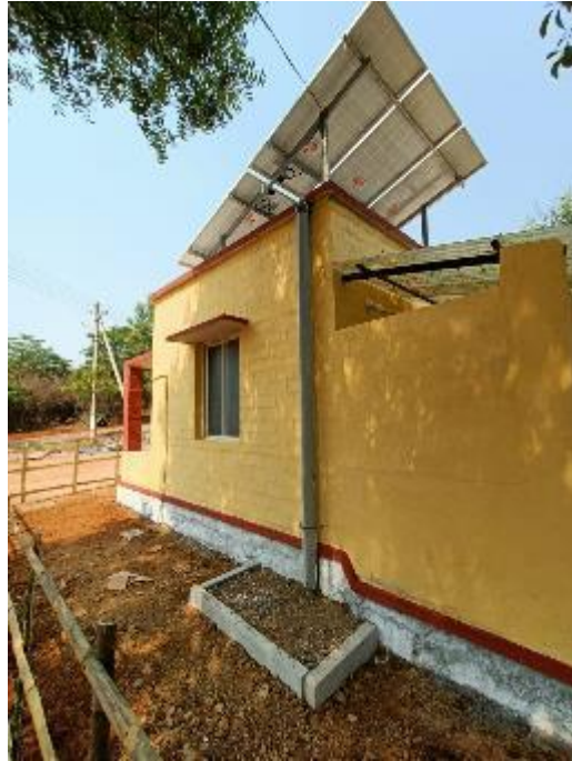
Roof Top Rain water Harvesting (Catch the Rain Program – Jal Sakthi Abhiyan-)
