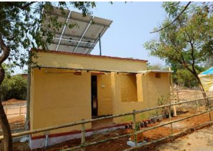
View from North
